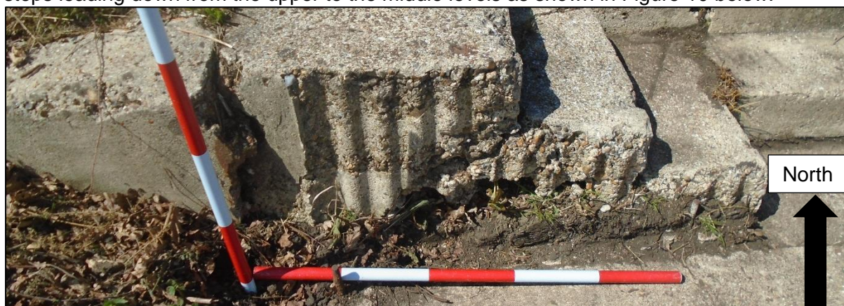
Figure 10: Evidence for corrugated wall construction in middle level of Ablutions Shed
