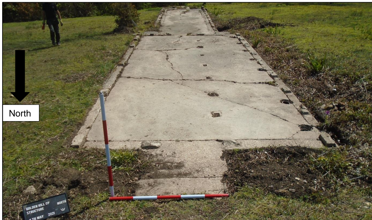
Figure 8: The upper level of Structure 1 the Ablutions Shed
