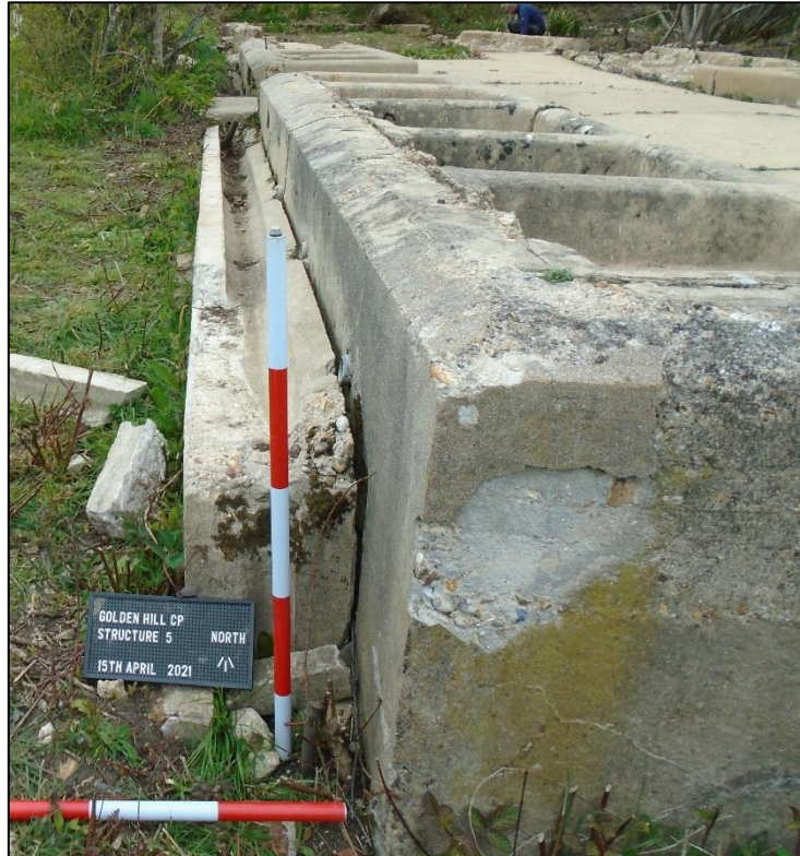
Figure 23: The outside waste water channel from the shower cubicles in Structure 5
