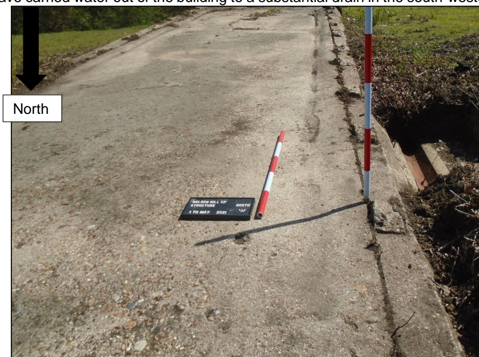
Figure 9: Middle level of the Ablutions Shed
